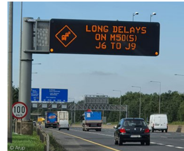
Figure 27 VMS displaying travel time message
