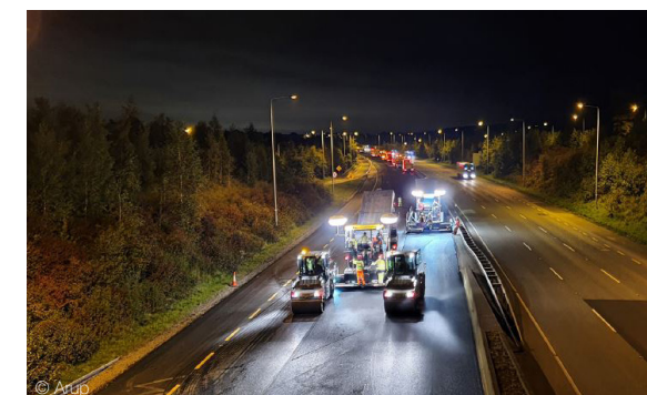
Figure 24 Maintenance of TII road pavement (17)
