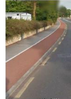
Detail 3 (photograph) is a possible option to be considered between ch 0+150 -ch 0+400 on the eastbound verge at detailed design stage which involves the widening of the existing footpath to accommodate both cyclists and pedestrians.
