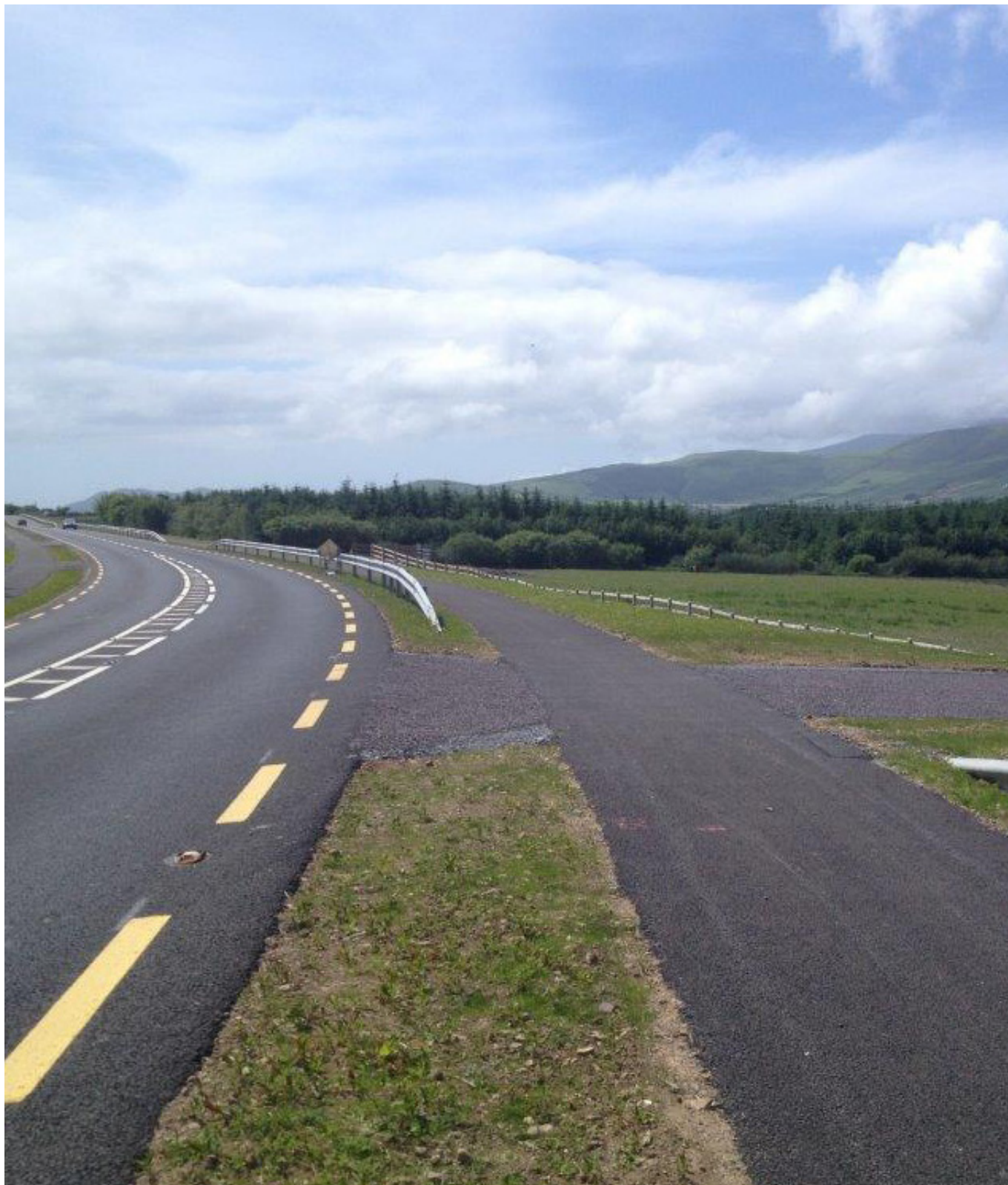
Figure 3 Segregated cycling/walking facility on N86 near Annascaul, Co. Kerry
